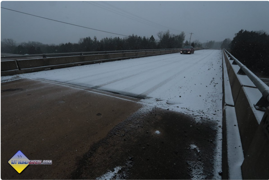
Fig 3b: Icy bridge in Bloomsdale, Missouri
