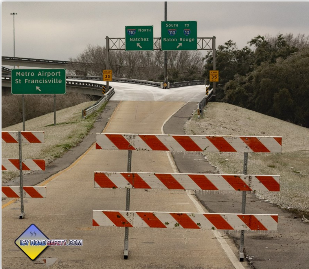
Fig 1b: Closed icy highway interchange in Baton Rouge, LA
