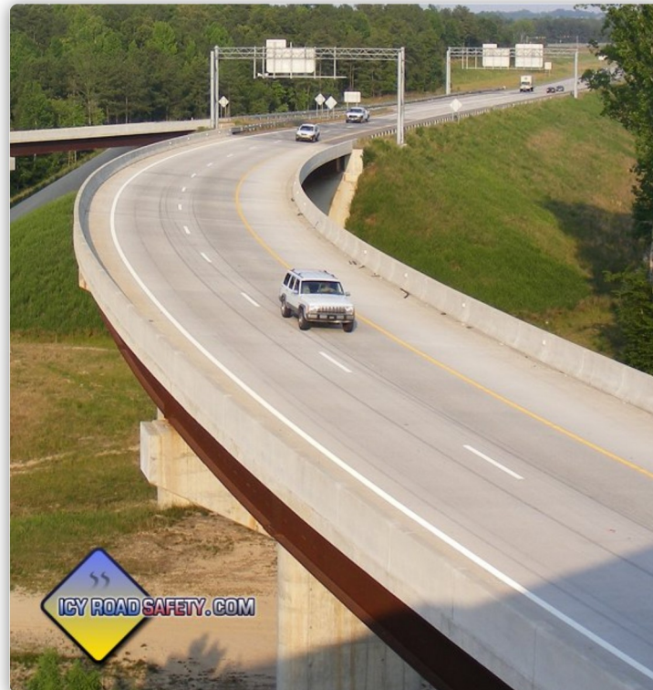
Fig 5h: Confining barriers are an inherent characteristic of every highway bridge.
