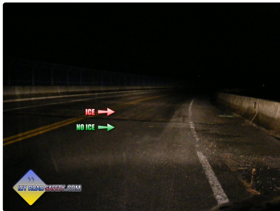
Fig 3h: Freezing rain icing on bridge near Beckley, West Virginia
